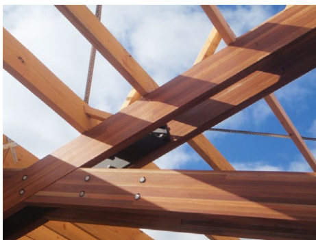
Figure 9. Engineered timber has become a primary structural component.
