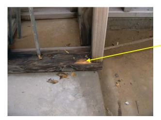
Although heavily discoloured with surface mould and blue stain, the pine timber is still sound as shown by scraping back the surface layer
