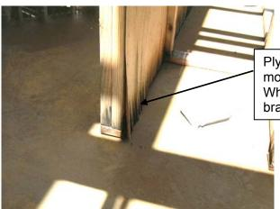
Plywood sheet bracing affected by moisture. Replacement required. Where necessary fix temporary braces.
