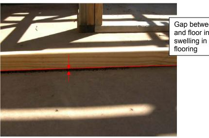
Gap between straight edge and floor indicates edge swelling in particleboard
